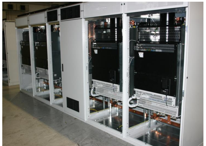
Fig. 2-3: Main DC Drives panel supplied by AIC and equipped with PowerFlex DC Drives
