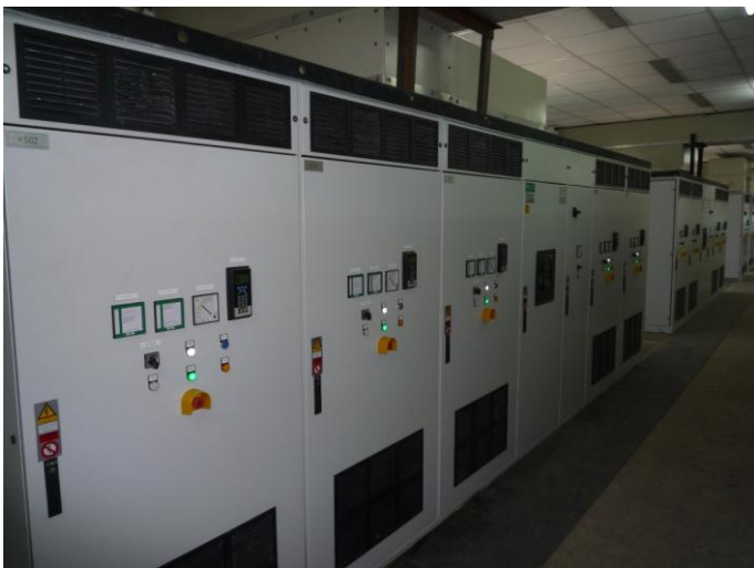
Fig. 2-3: Main DC Drives panel supplied by AIC and equipped with PowerFlex DC Drives
