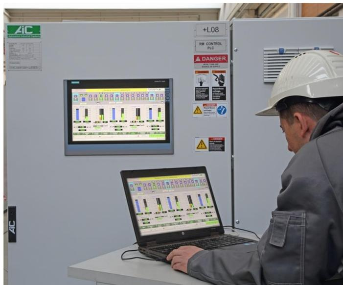
The panels are carefully designed to reduce as much as possible the risk of arc flash with several active protections; two systems were implemented to prevent the risk of arc flash:
